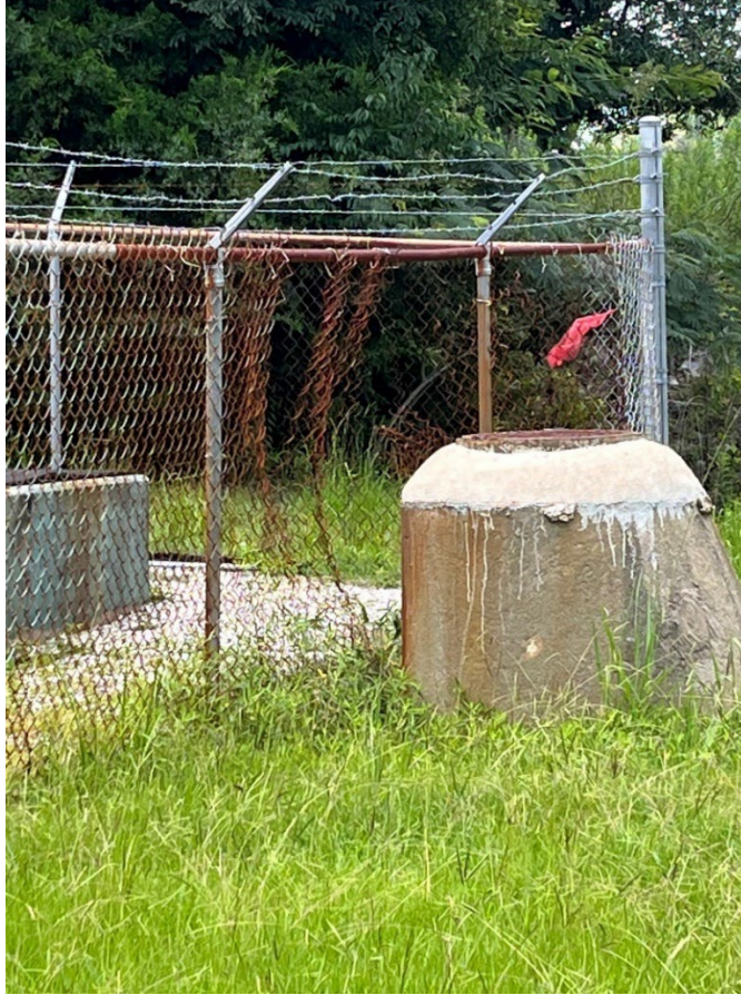
Fence hole at Lift Station 42. Taken July 18, 2023.
