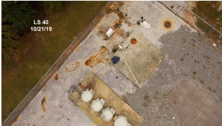
Aerial view of Lift Station 40. Taken Oct. 21, 2019, by John Wathen, Hurricane Creekkeeper.
