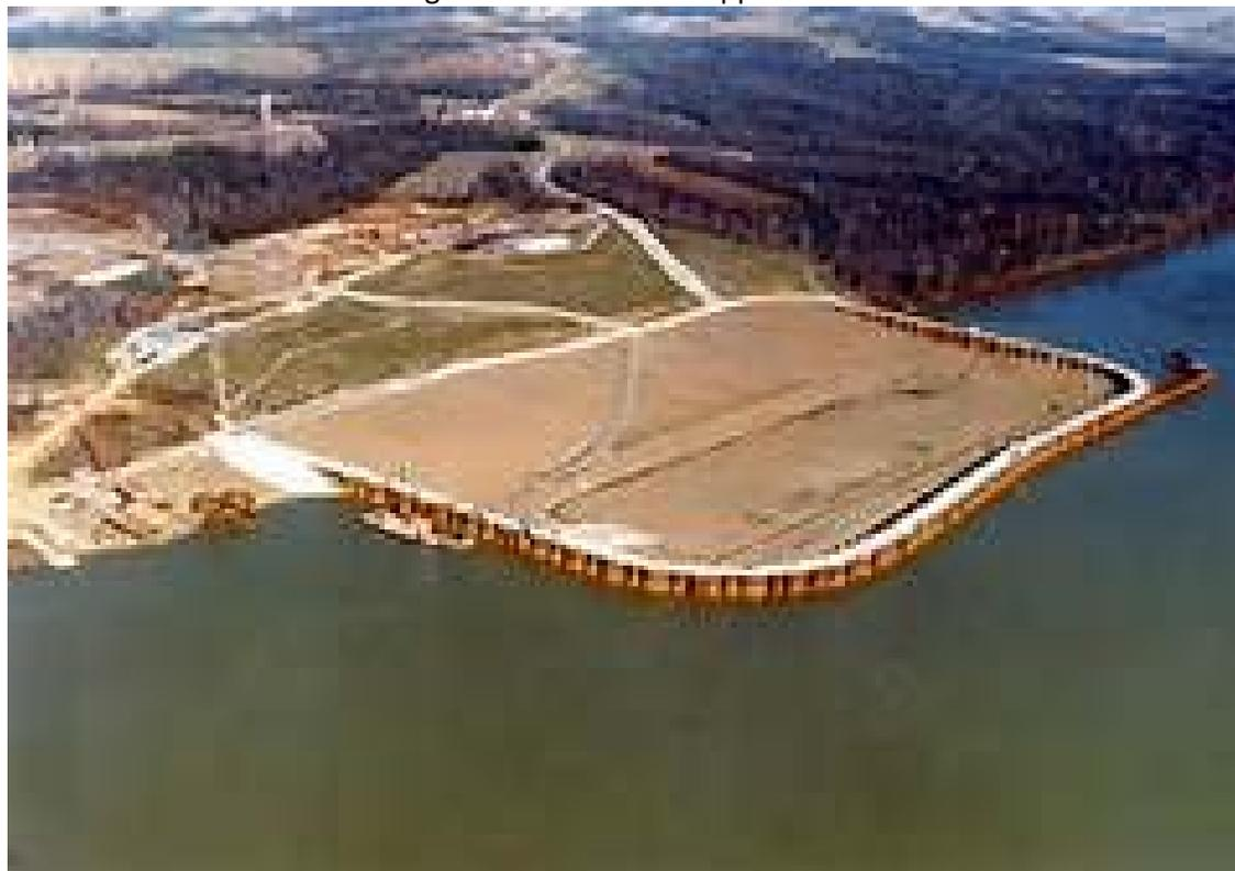
The following photos show a coffer dam that was constructed in a river upstream of a main dam at the Merian Mine Site in Suriname South America for Newmont Mining Corporation. In the second photo the cofferdam is to the left of the large orange Hitachi excavator. The cofferdam was constructed to prevent stormwater runoff water and seepage water from flowing into the dam work area. The contained water was then be pumped downstream of the work area.
