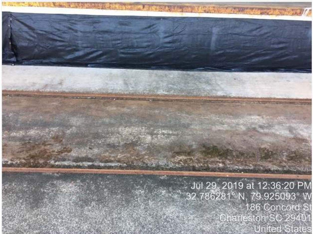
Rail track and silt fencing
