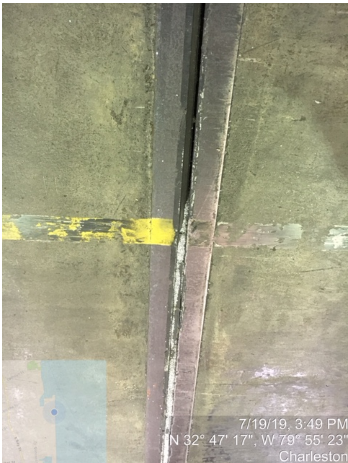
IMG_1785 – INSIDE FACILITY – SEAM WITH PLASTIC ACCUMULATION IN POOR REPAIR – SEAM OVER WATER
