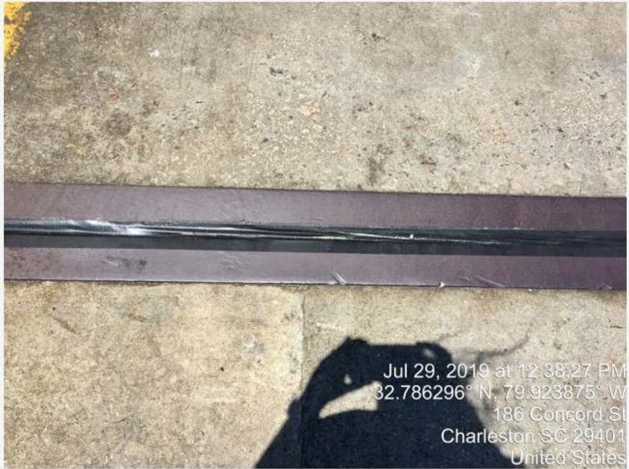
Expansion joint covered with tape
