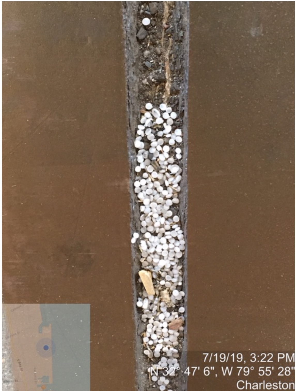
IMG_1779 – INSIDE FACILITY – DETAIL OF PLASTIC ACCUMULATION ON COVERED SEAM
