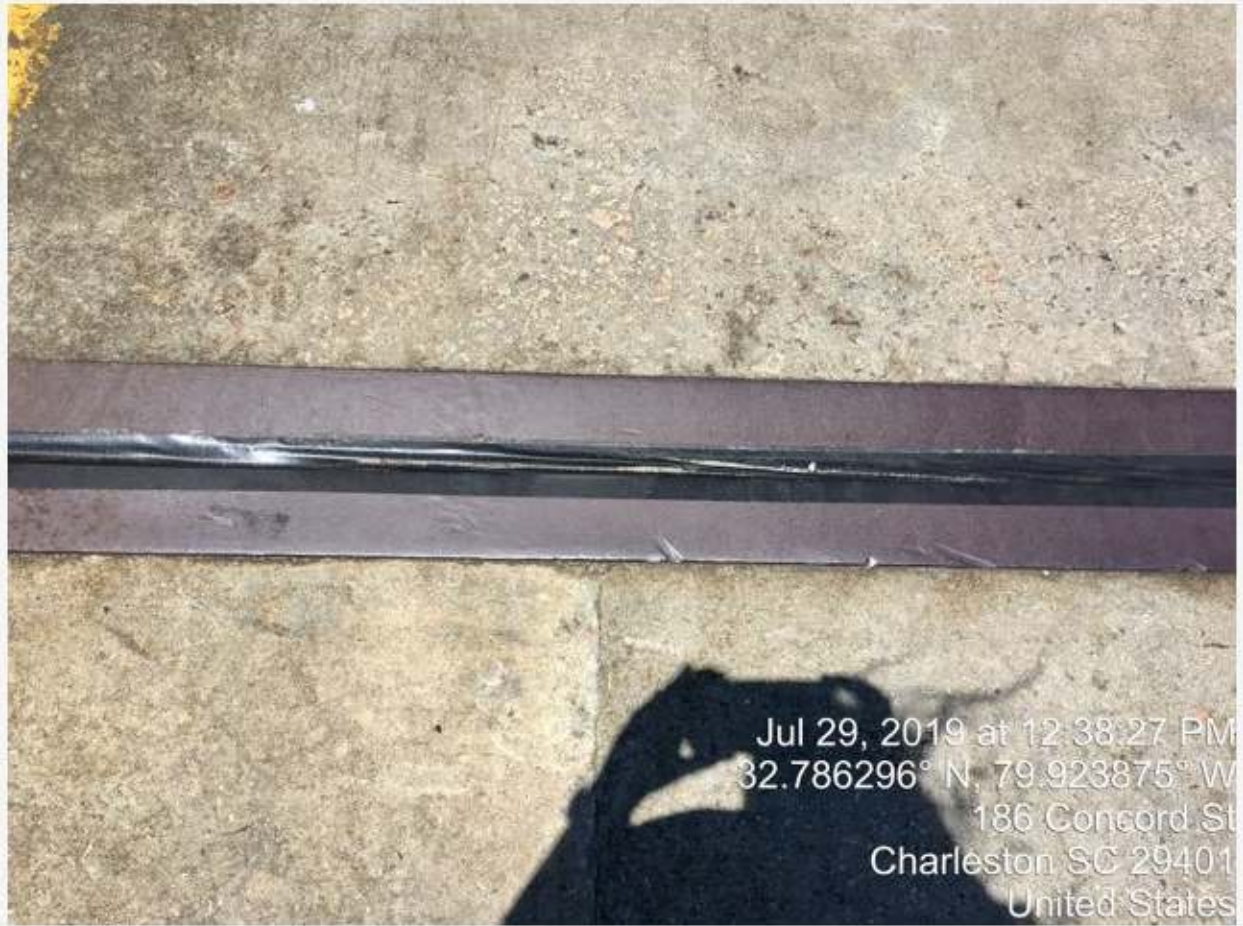
Expansion joint covered with tape
