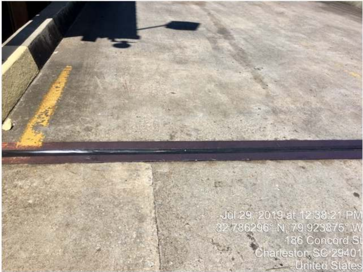
Expansion joint covered with tape 2
