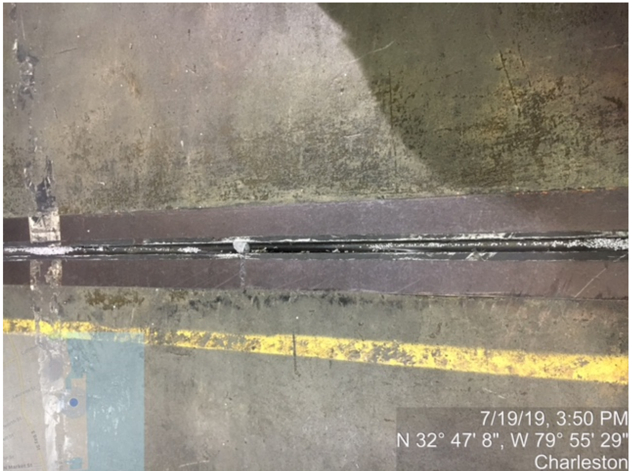
IMG_1787 - INSIDE FACILITY - SEAM WITH PLASTIC ACCUMULATION IN POOR REPAIR – SEAM OVER WATER
