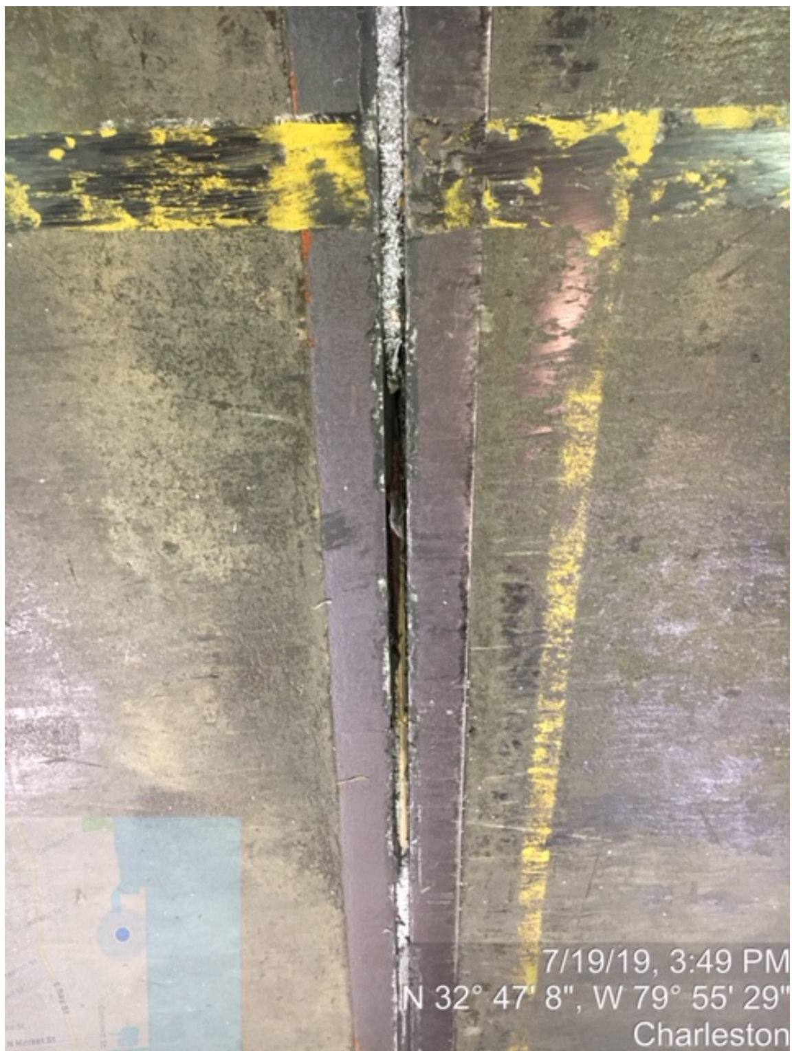
IMG_1786 – INSIDE FACILITY - SEAM WITH PLASTIC ACCUMULATION IN POOR REPAIR – SEAM OVER WATER
