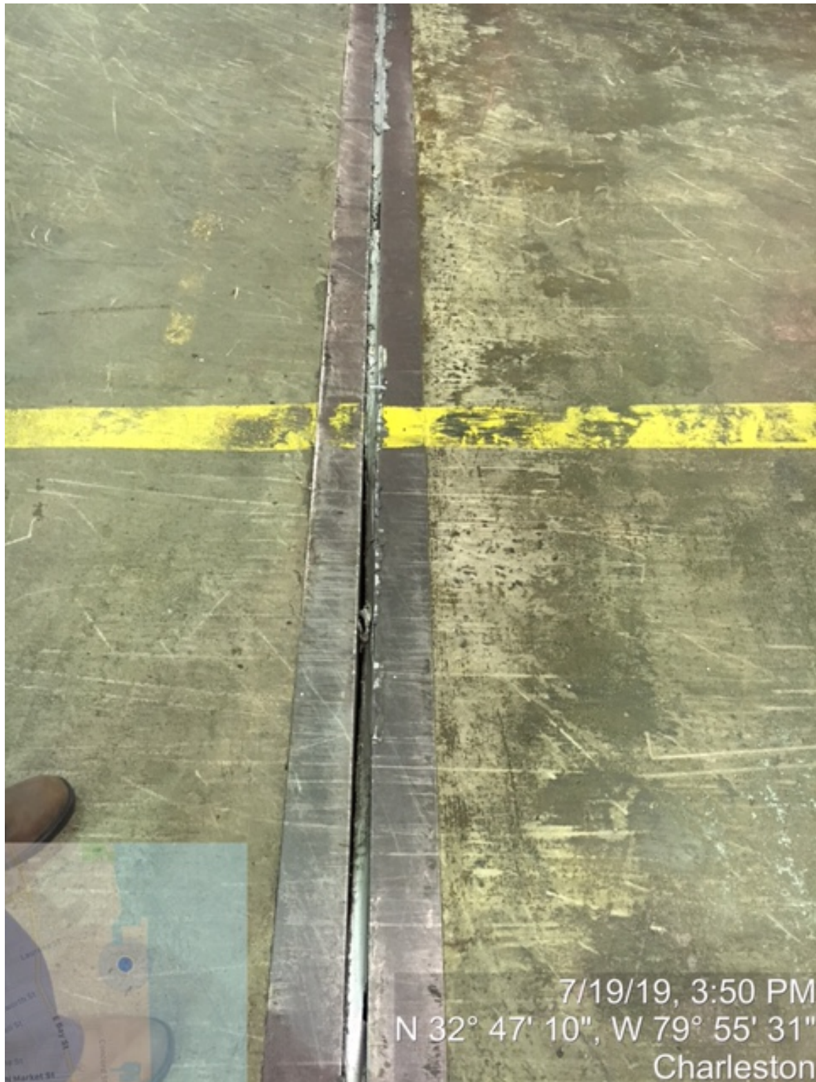
IMG_1788 - INSIDE FACILITY - SEAM WITH PLASTIC ACCUMULATION IN POOR REPAIR – SEAM OVER WATER
