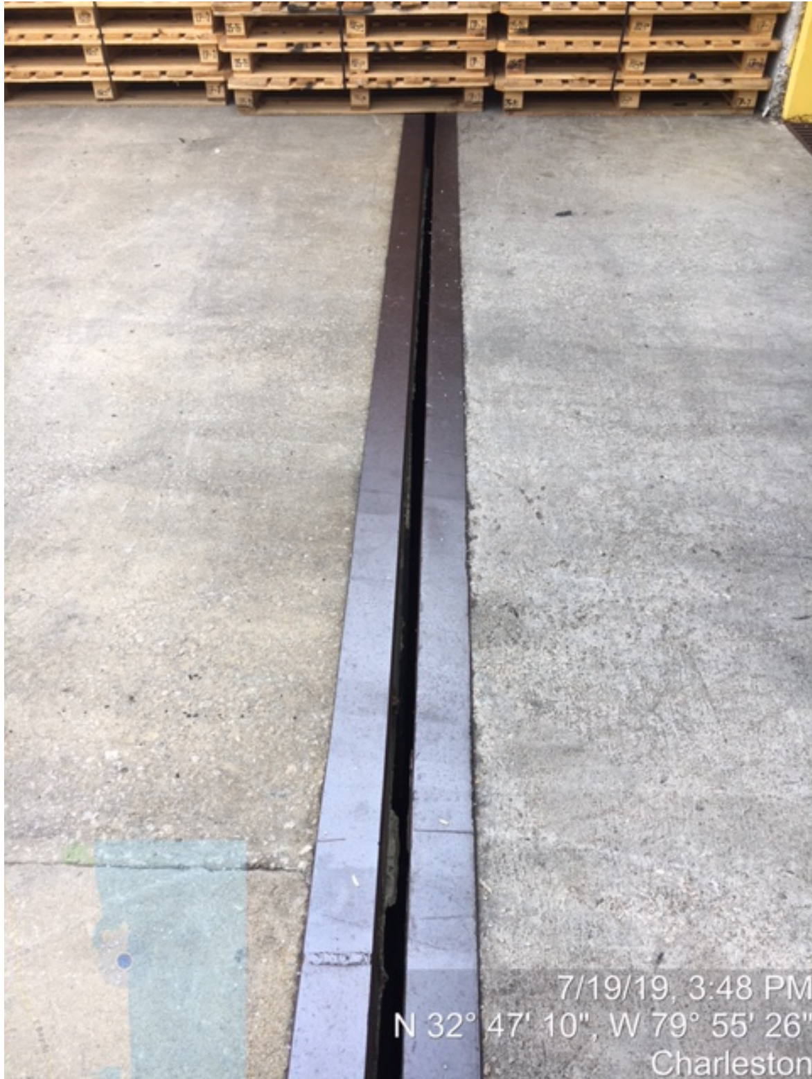
IMG_1783 – BACK DOCK AREA - EXPOSED SEAM BETWEEN BACK DOCK AREA AND FACILITY
