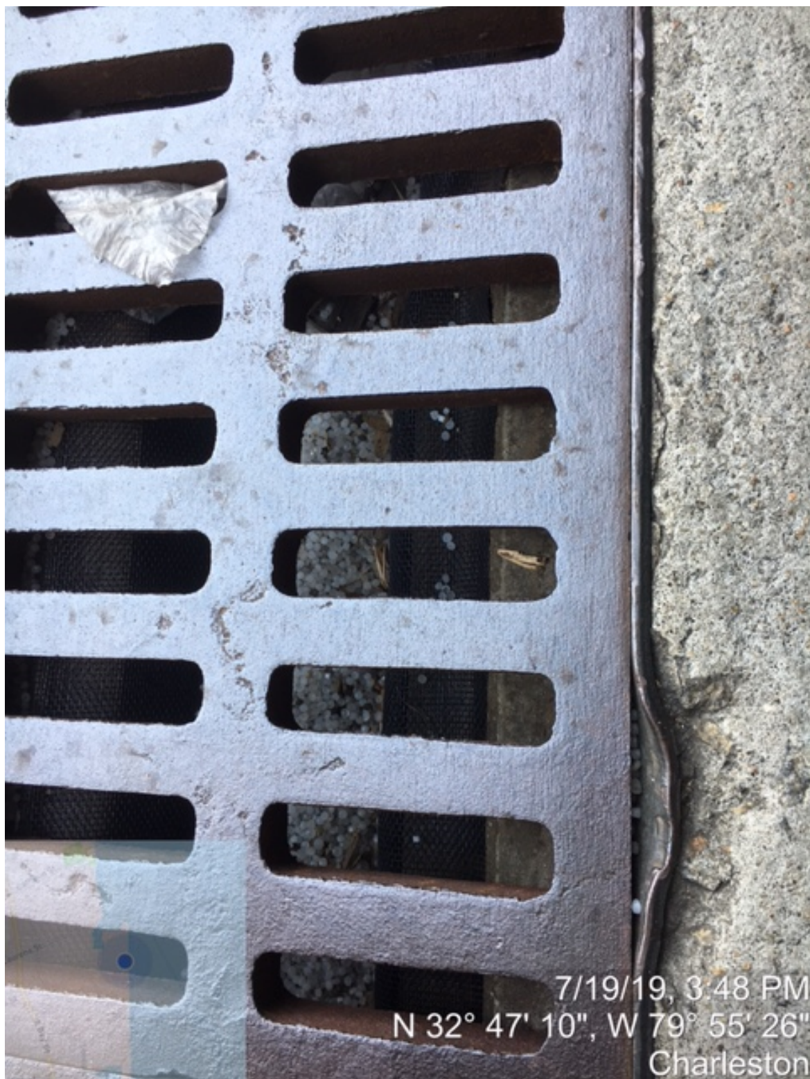
IMG_1782 – SCREENED GRATE AT FACILITY BACK ENTRANCE
