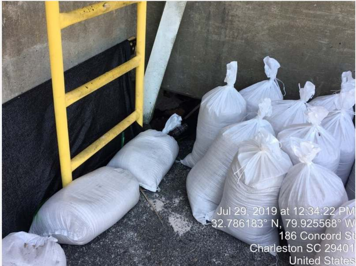
Gap in silt fencing by seawall
