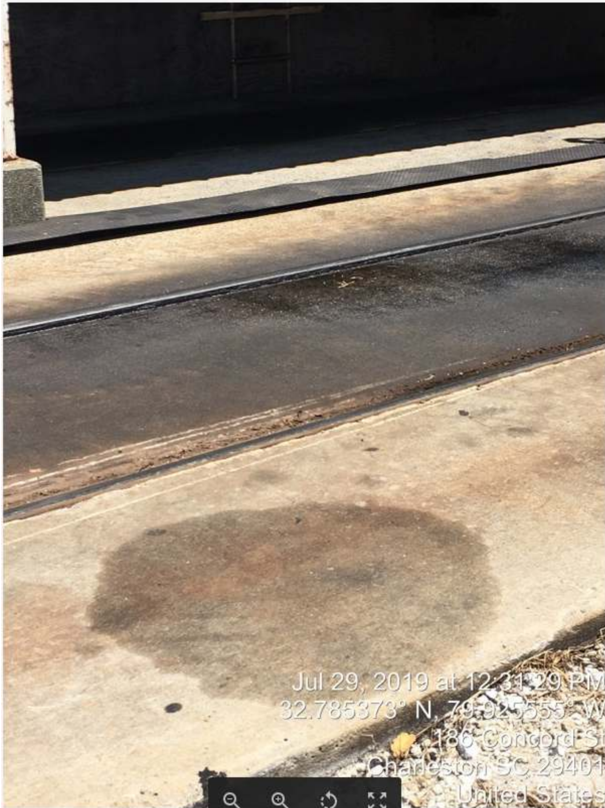
oil spillage on rail track
